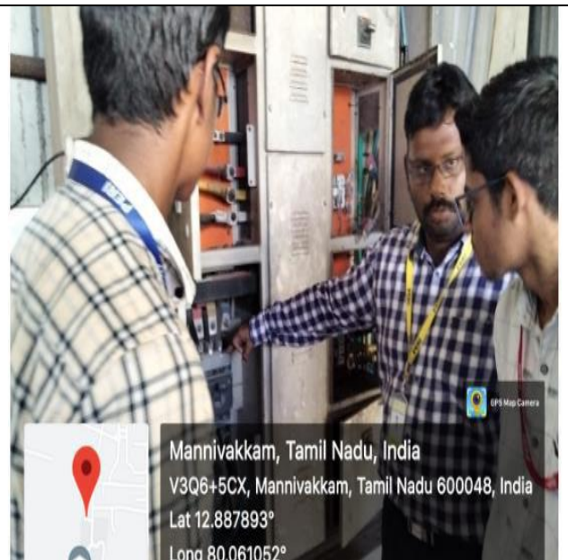
EEE students getting information about wiring of transformers connections
